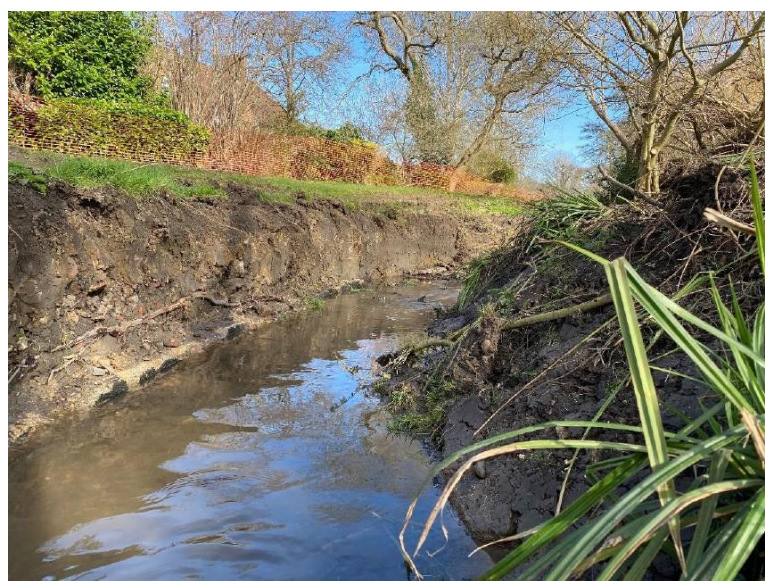
Figure 5-2 Riverbanks of the Burnt Oak Brook after concrete removal Image Credit: Unblocking the Burnt Oak Brook Project Report, Thames21
