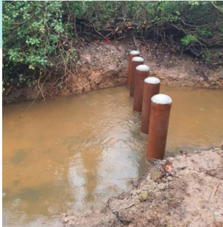
Figure 6-6 Trash pins at Southover Image Credit: Barnet Council
